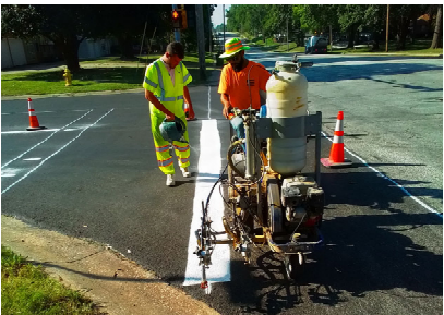
Pavement Marking Project
