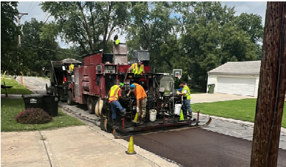
Modified Aggregate Quick Set (MAQS) Resurfacing Project
