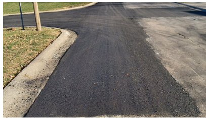
Asphalt Street Patching
